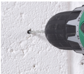
Drill a 5mm pilot hole
