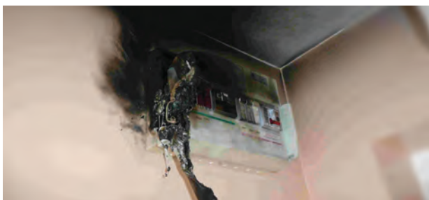
Result of a DIY home owner having wired an 10.5 kW electric shower circuit with 2.5 mm 2 cable and a 45 A circuit-breaker. (Photo courtesy of British Gas)
